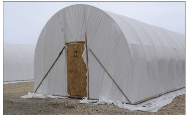
Figure 3. Poly-covered Quonset-type greenhouses are used for winter protection of container grown plants.
